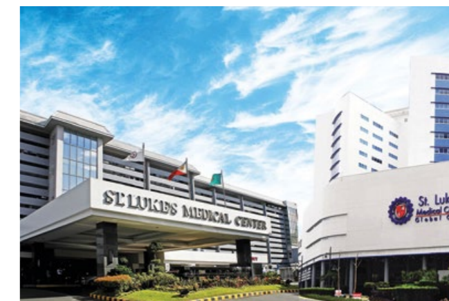
St. Luke’s Hospital, Metro Manila, Philippines
